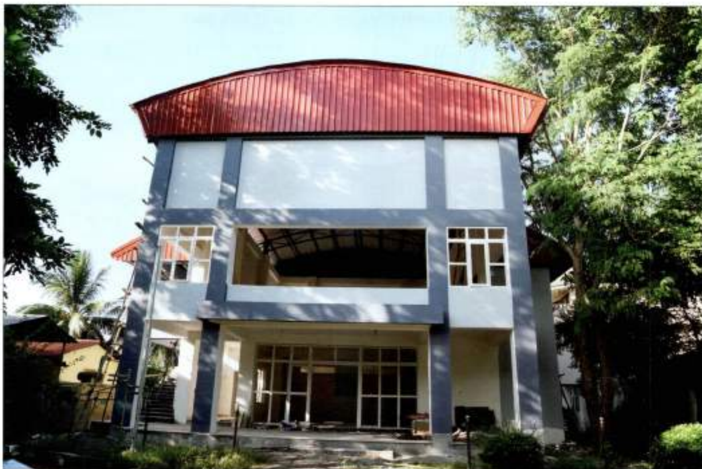
Sports Facility building for Gymnasium, Badminton and Table tennis
