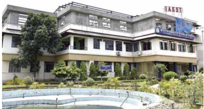
View of the vertical extension work over the Library building
