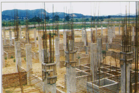
CONSTRUCTION OF IASST - COMPLEX IS IN PROGRESS.
