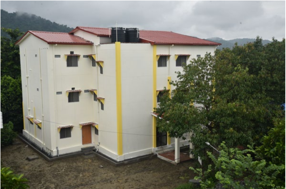
SC/ST training facility getting complete
