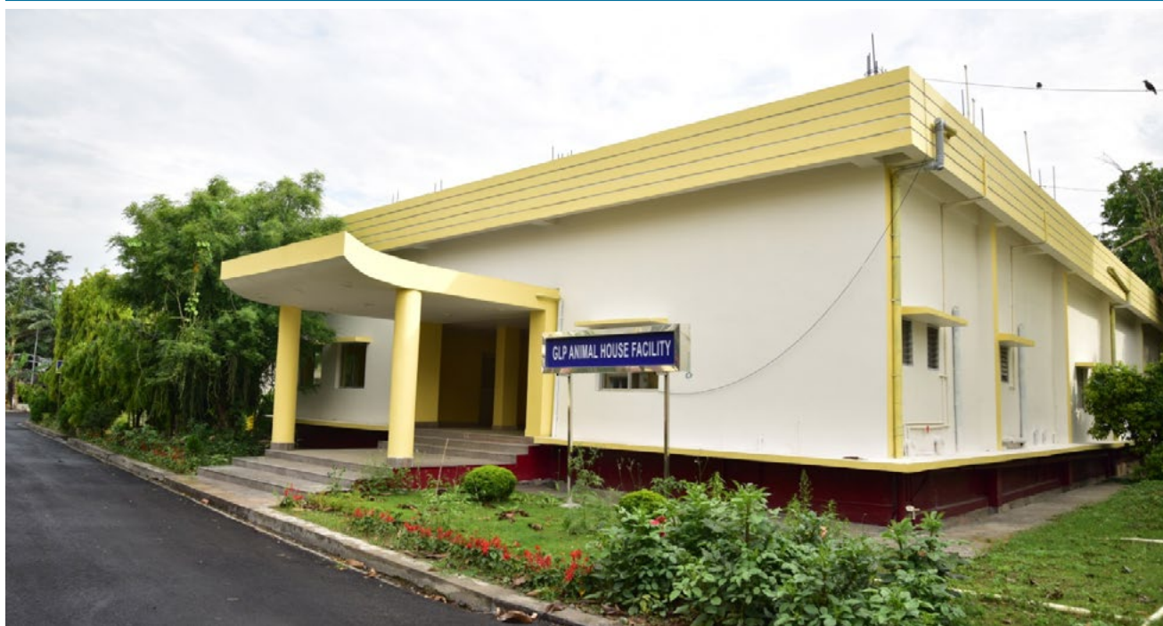
Front view of the Animal House Facility building
