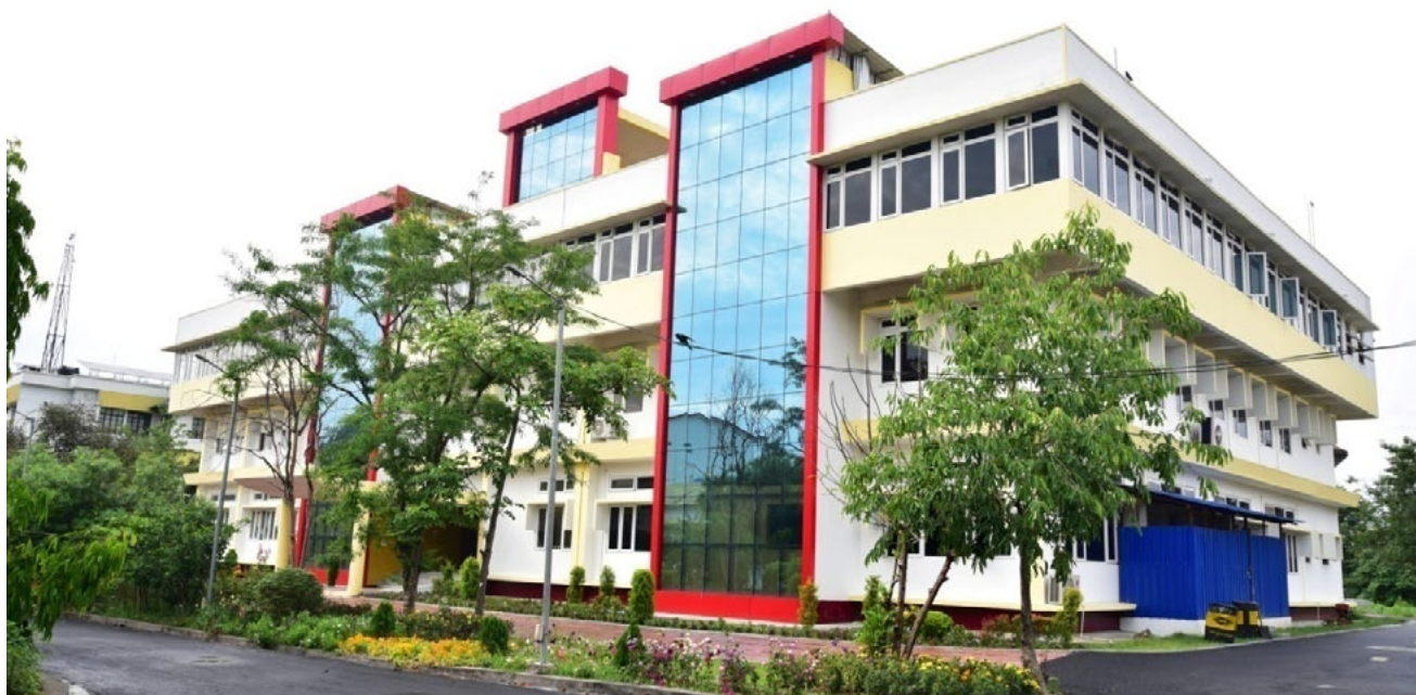
A view of the newly constructed Central Instrumentation Facility (CIF) building
