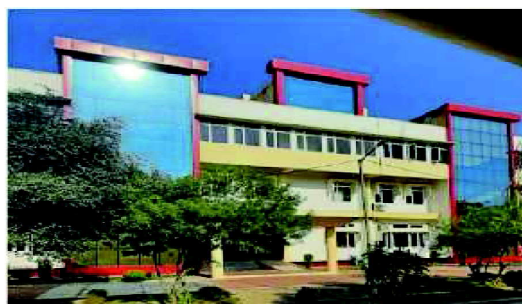
Bionest-IASST is housed in 2 nd floor of SAIC building.
