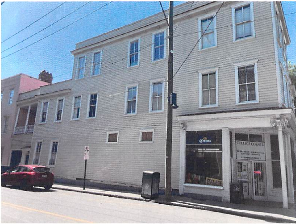
Additional Figure #19: Image of the South Elevation
