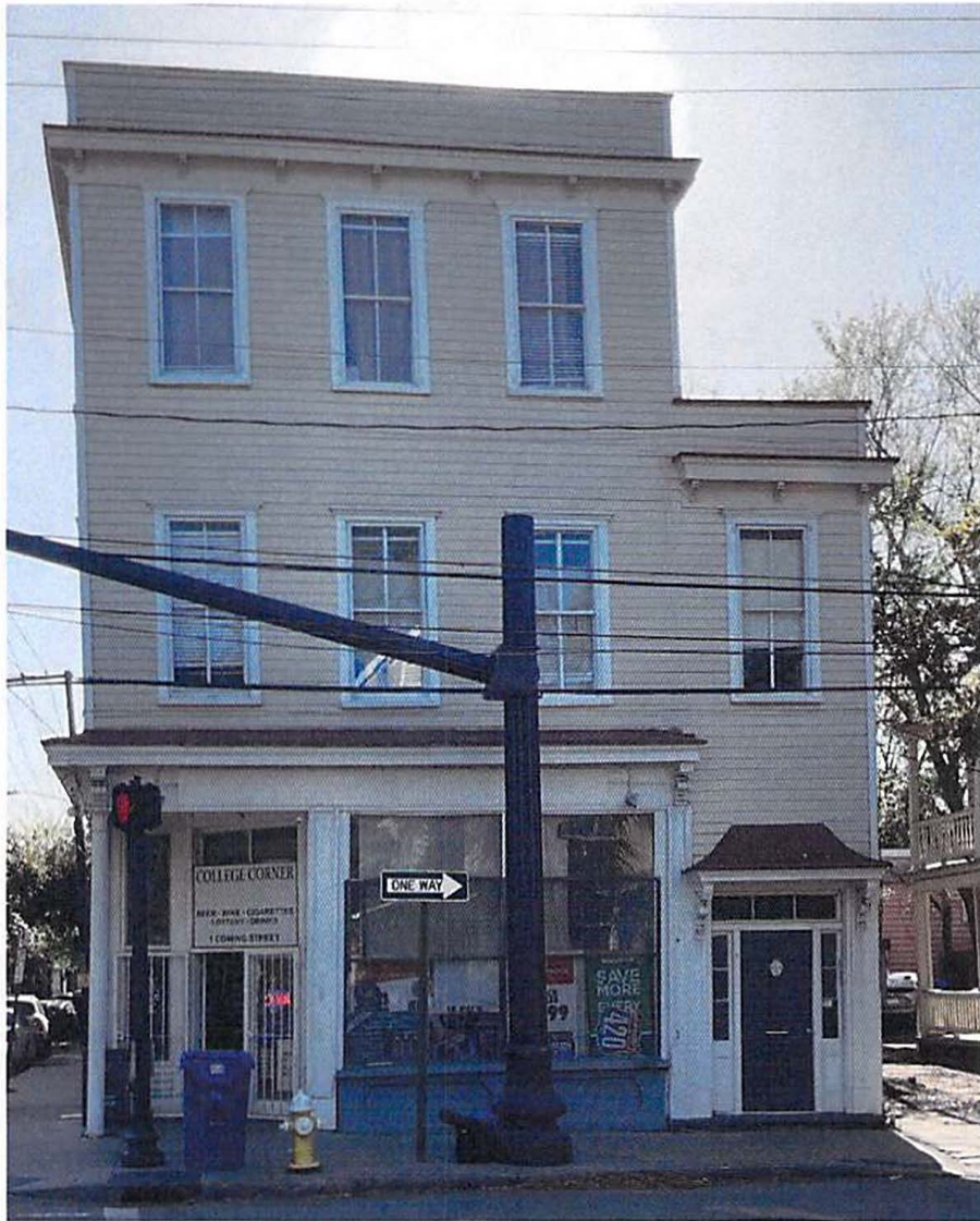
Additional Figure #17: View of the East Elevation
