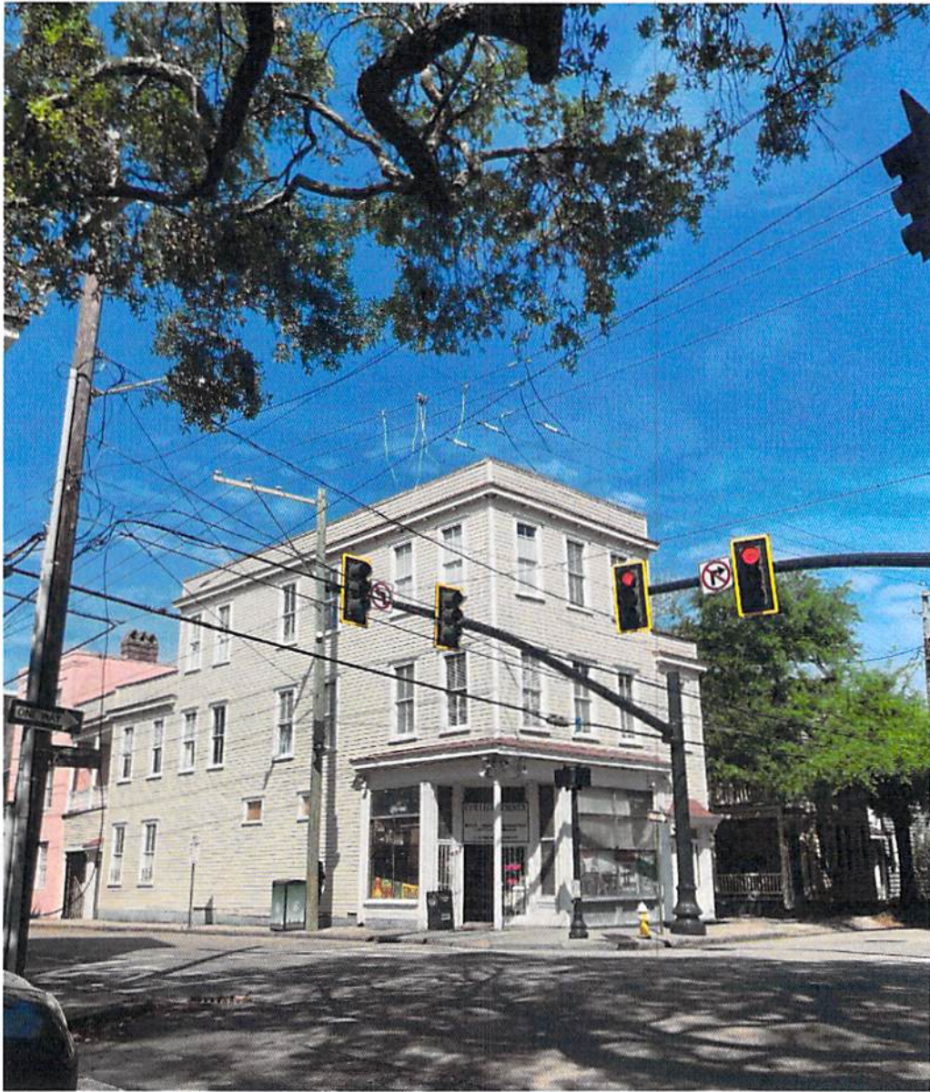
Additional Figure #18: View of the Southeast Corner
